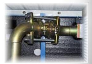
One connection to the separator vessel
